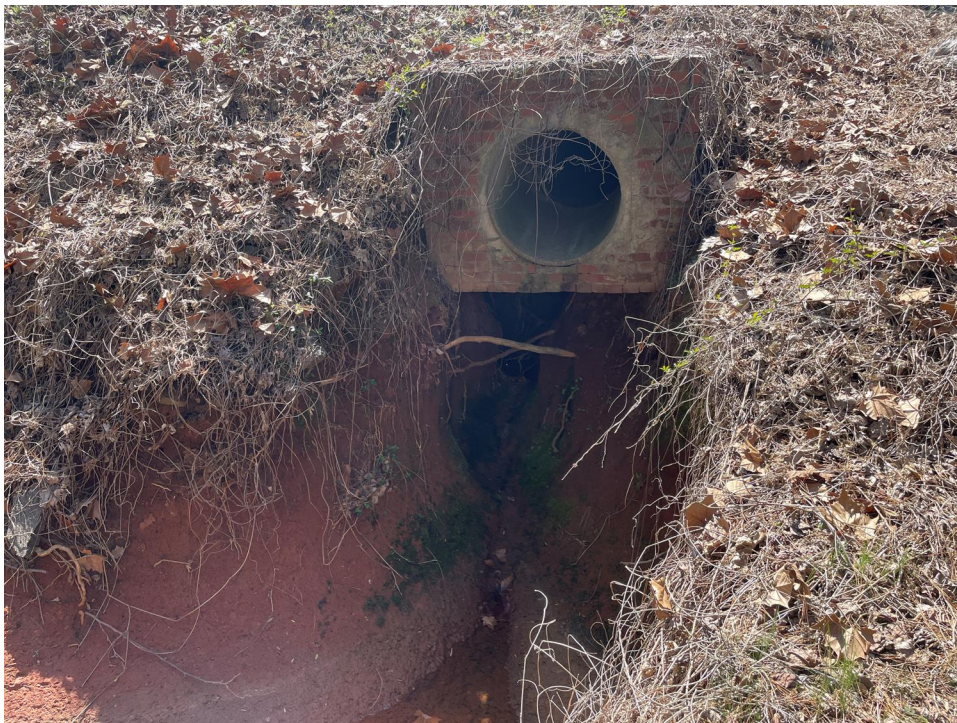
Figure 3 - Erosion below stormwater outfall conveying water from Ryerson.
