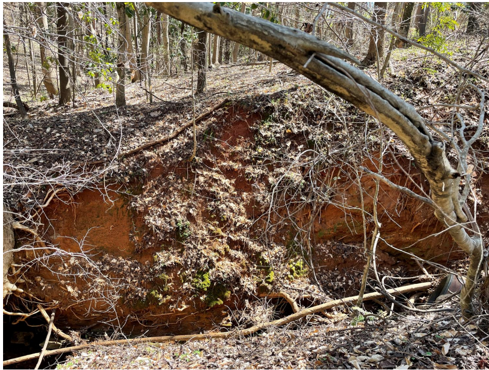
Figure 4 - Example of severe erosion below outfalls in Pond A.
