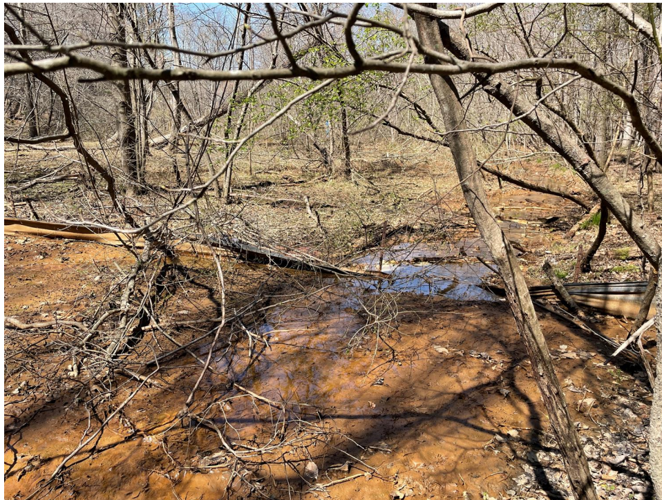
Figure 6 - Sediment deposited in wetlands adjacent to silt fence.
